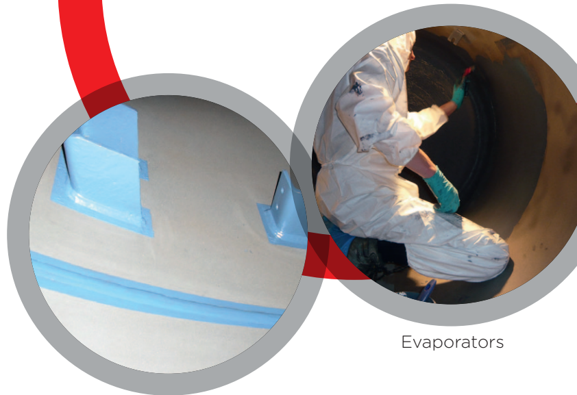
Welds and Brackets
