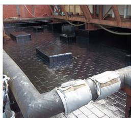
Static dissipative and chemically resistant coating for primary and secondary chemical containment areas including bunds, drains, sumps and channels.
