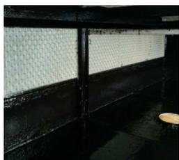
Static dissipative and chemically resistant coating for fuel storage tanks and hydrocarbon tanks where fluid is agitated (i.e. pumping and piping and filtration systems).
