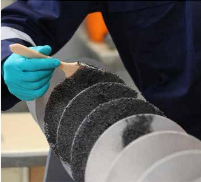
Belzona 1814 is a cost-effective three-component repair system for the protection of surfaces subject to abrasive attack.
