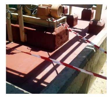
Belzona 4131 (Magma-Screed) is a two-component system for the repair and resurfacing of concrete and stonework.
