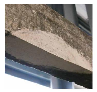
Belzona 4141FR is a fire-resistant, lightweight repair composite for the rebuilding and protection of damaged vertical and overhead concrete surfaces.
