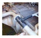
Belzona SuperWrap II is intended for use on various geometries of pipes, including bends, straights, tees, reducers and flanges.
